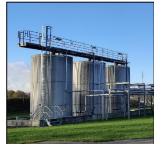
Pictures from O8 Oils Storage Facility at Aarhus Havn (DK), Yara Lye Storage Facility at Vejle Havn (DK), and an API Ethanol Storage (DK)
